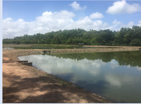
Figure 22: Hikkaduwa Sewage Treatment Plant
