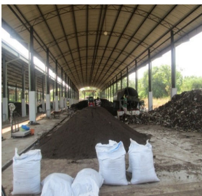
Figure 5: Composting Facility at Keerikkulama (Anuradhapura)
