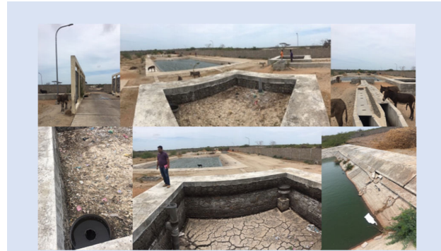
Figure 38: Septage treatment plant in Mannar
