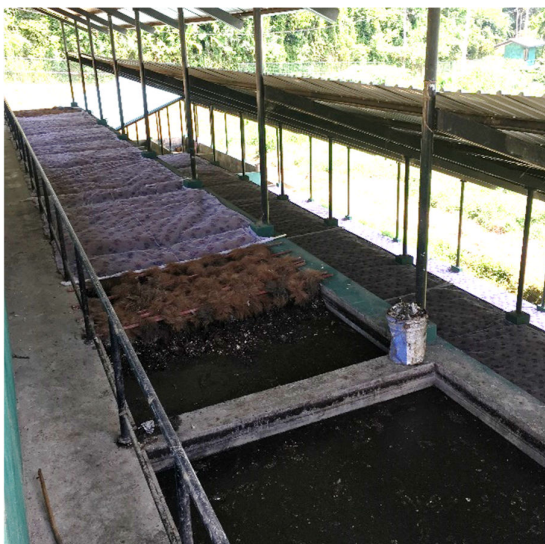
Figure 62: Septage treatment plant at Kanadola
