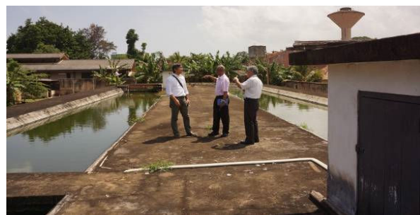
Figure 42: Water Treatment Plant (Matara MC)
