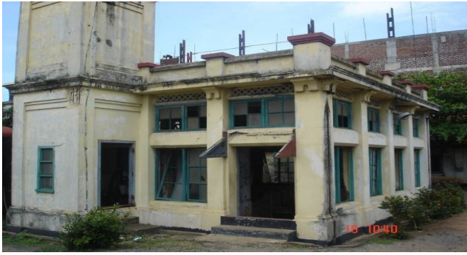
Figure 17: Pumping station (Bambilapitiya) Source: CMC
