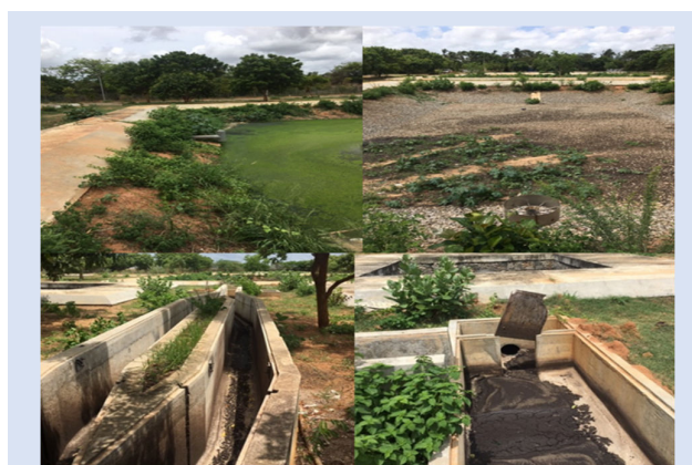
Figure 58: Septage treatment plant in Puttalam
