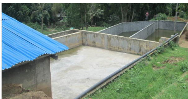
Figure 28: Kandy Septage Treatment Plant
