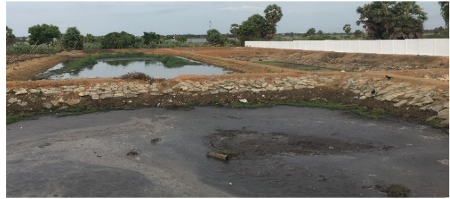
Figure 10: Batticaloa MC Septage treatment plant Photo credit: IWMI
