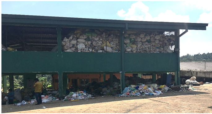
Figure 59: Plastic and polythene recycling centre at Kanadola
