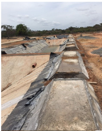
Figure 31: Construction of the new STP – Kilinochchi (photo credit: IWMI)
