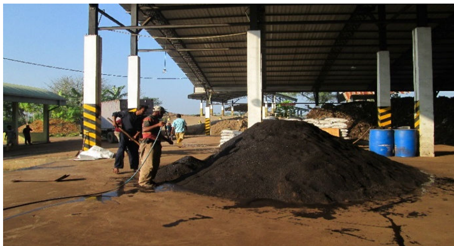
Figure 26: Composting facility at Pohorawatta
