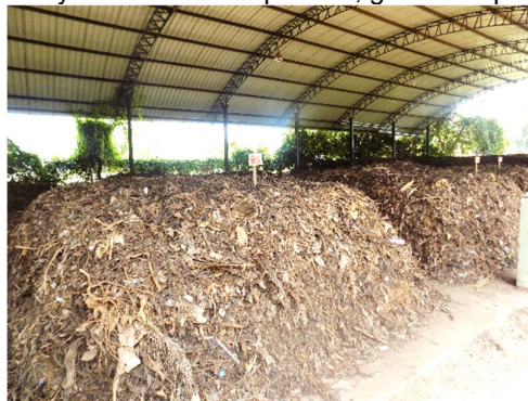
Figure 48: Negombo MC Compost plant (photo credit: IWMI)
